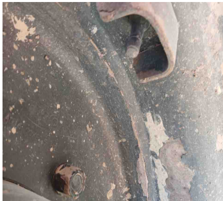
Wheel Position: A1 - Damage Size
